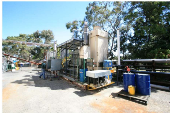
Engine and generator running on Syngas
