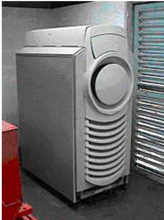
Photograph 2. Capstone micro-turbine in the engine house
