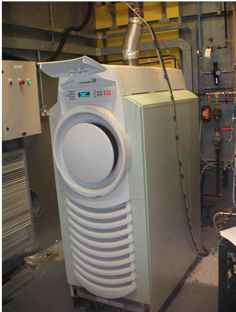
**Figure 10: Capstone Microturbine in Advantica Test Cell 2**
